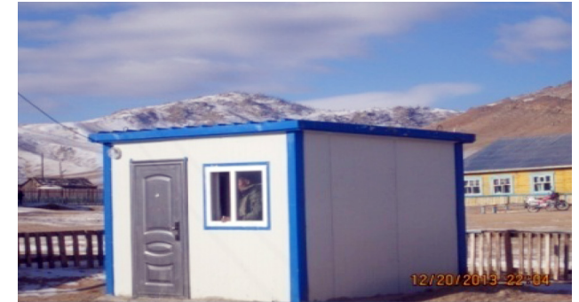
The school deep well, Burentogtokh
