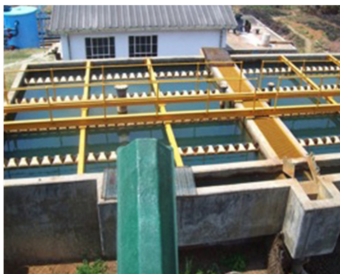
New water pumps (left) installed at Shurugwe water treatment plant and rehabilitated sedimentation tank (right) at Chipinge water treatment plant
