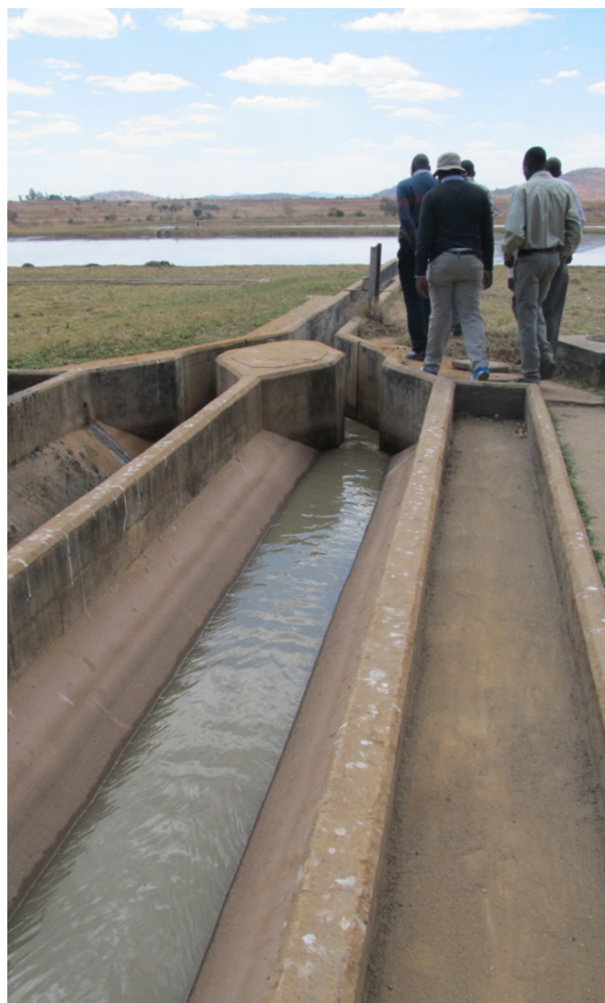
Bindura. sewage treatment ponds
